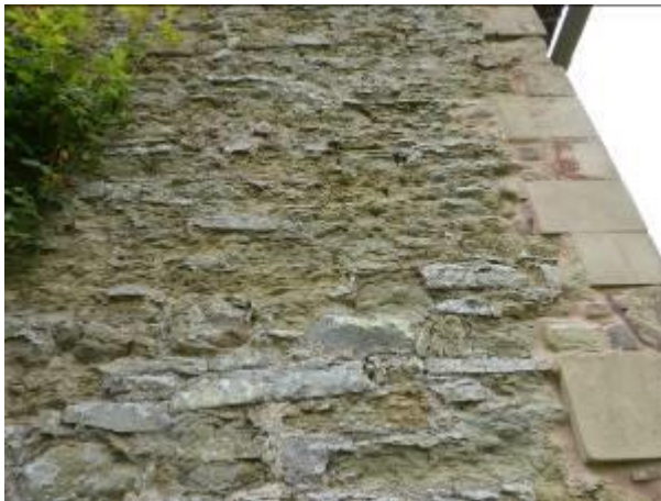
Nave west gable – Eroding stonework.
