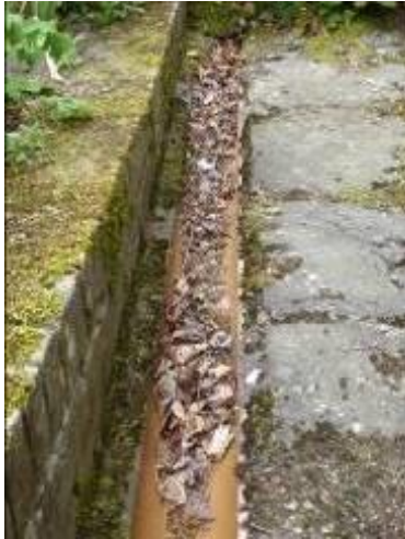
Drainage channel – Debris in channel.
