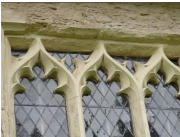
Chancel south – Damaged stonework to east window.
