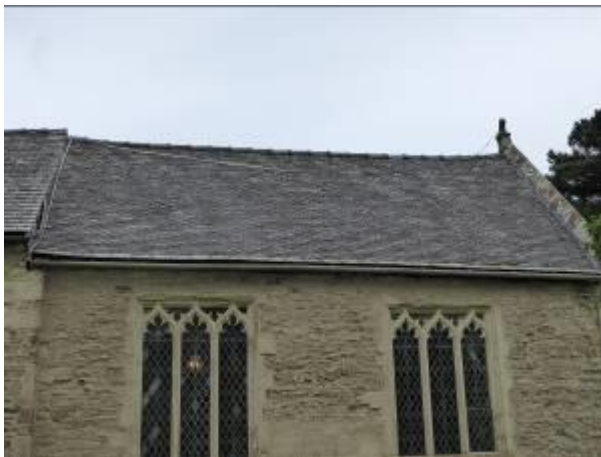
Chancel south – Poorly aligned gutter.
