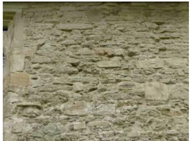
Nave south – Eroding stonework and open joints.
