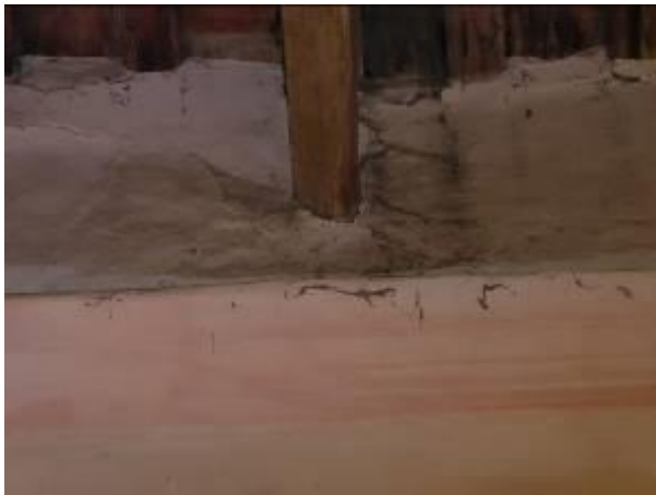
Nave roof – Damaged plaster above moulded cornice.
