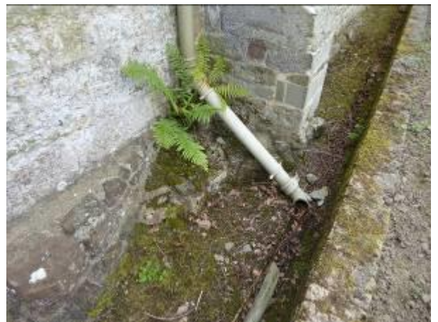
Chancel north – Poor rainwater disposal.
