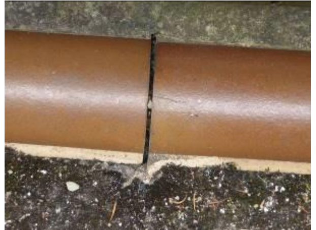
Drainage channel – open joints.
