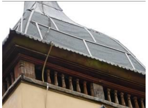
Turret roof – Temporary felt covering.
