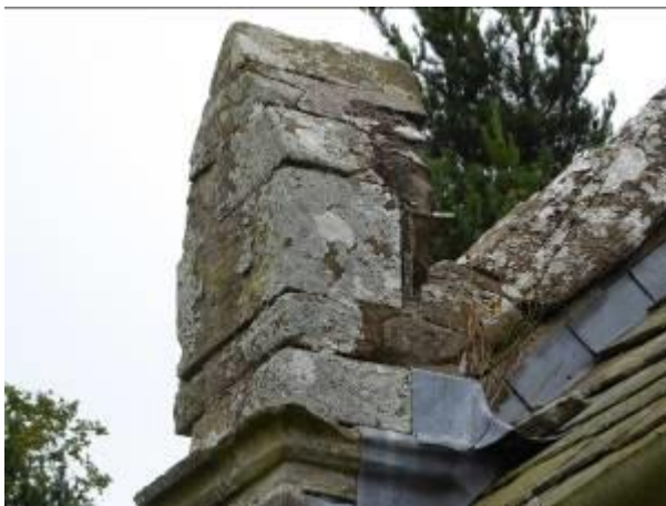
Chancel north east gablet – Open joints and heavily eroded stonework.
