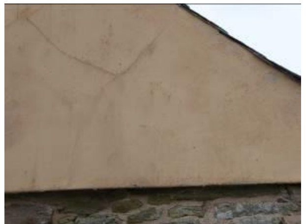
Nave west gable – Cracking to render.
