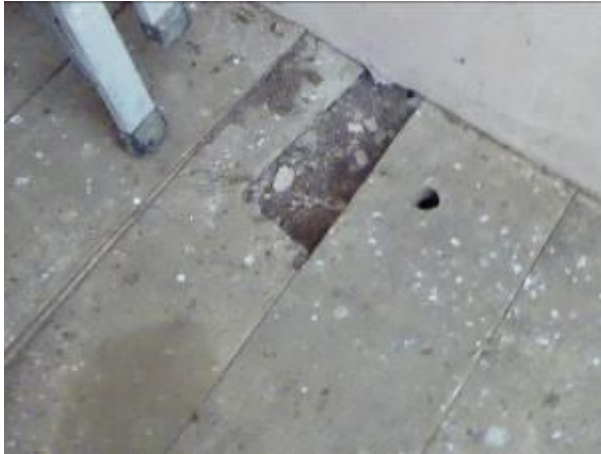
Turret first floor – Decayed and damage to floorboards.
