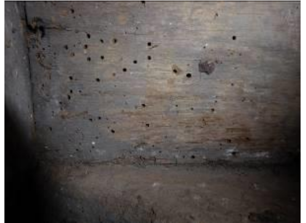
Turret interior – Wood boring insect activity.
