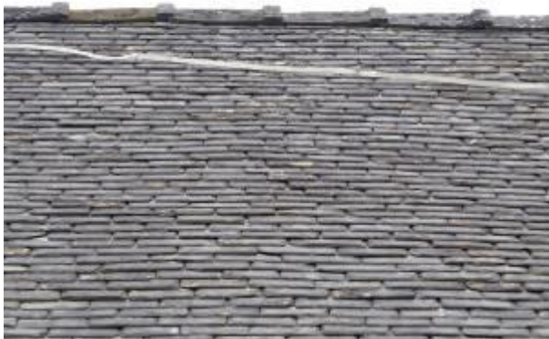
Lighting conductor – Slipped and dislodged.
