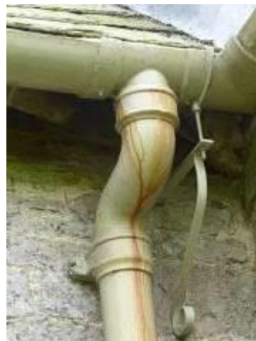
Chancel north – Rust staining to downpipe.
