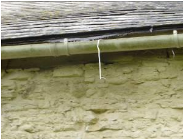
Nave south – Deteriorating roofing felt at eaves.
