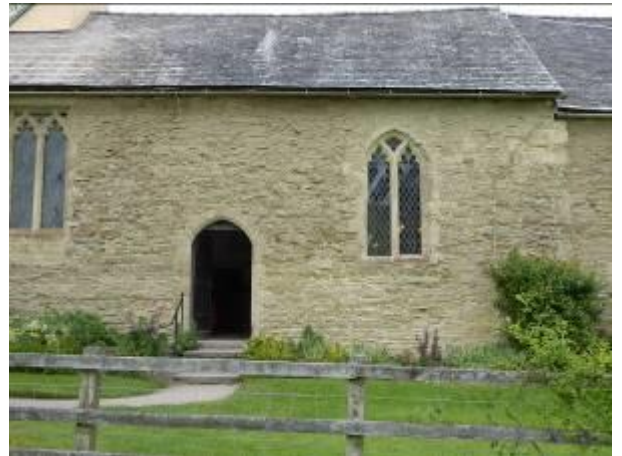
Nave south – Poorly aligned gutter.
