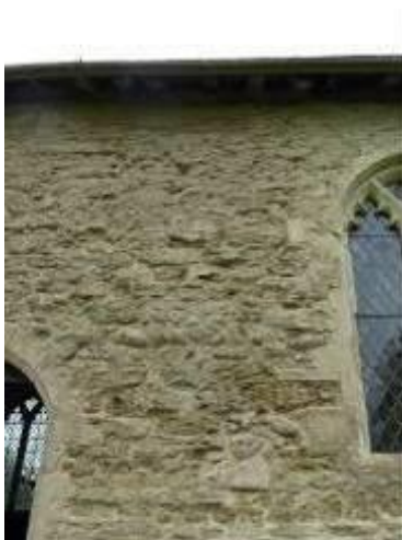
Nave south – Eroding stonework and open joints.
