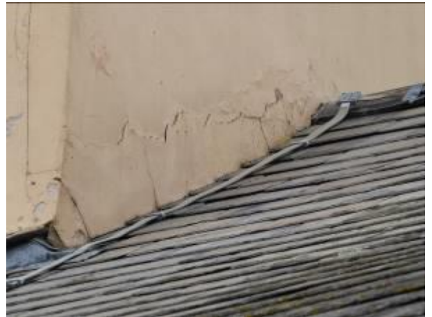
Turret east – Cracking to render over flashings.
