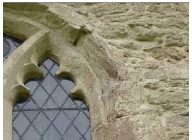
Nave south, east window – Damaged voussoir.
