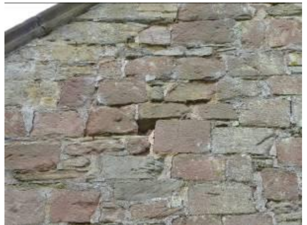
Chancel east gable – Open joints and voids.
