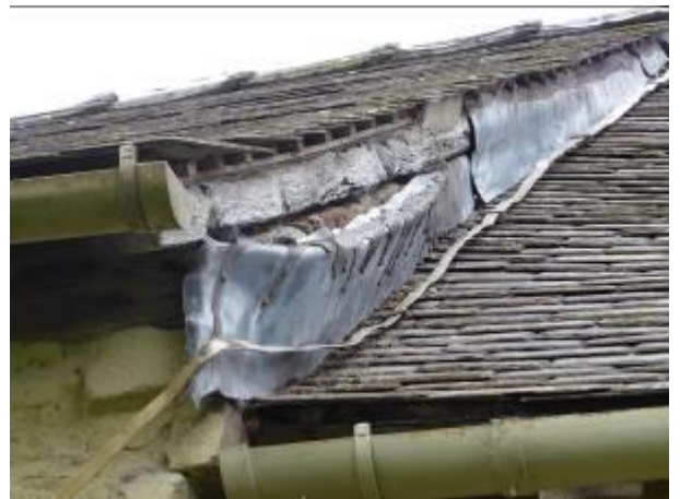
Chancel – Dislodged flashing at nave east gable abutment.
