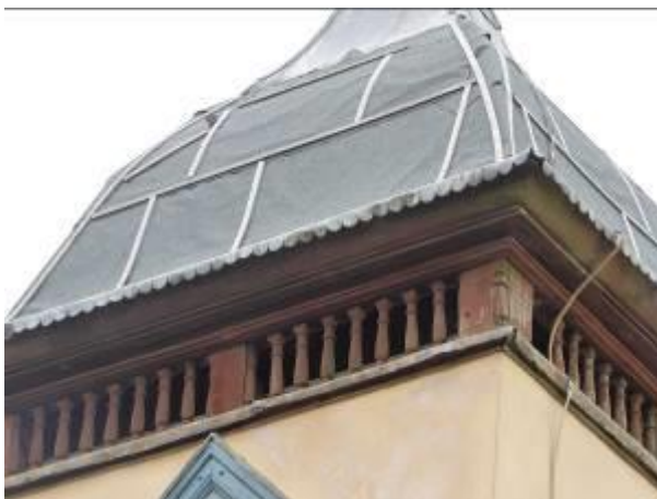
Turret roof – Temporary felt covering.
