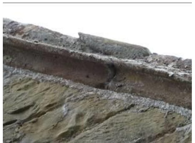
Chancel east gable parapet – Fractured moulding to coping.
