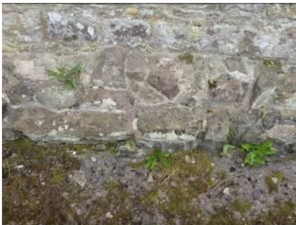
Drainage channel – Cracking to concrete at junction with external walls.
