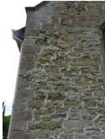
Chancel east gable – Open joints and eroding stonework.
